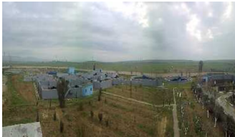
Photo 5 - La station d'épuration de SBA (ONA, 2015)
