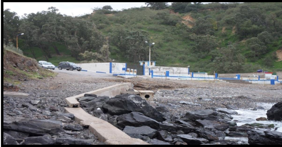
Figure 53 - Station de Pompage (Ghazaouet).
