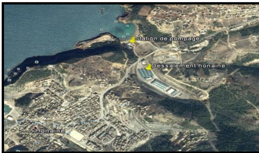
Figure 51 - Station de dessalement de Honaine [ Image Landsat 2015 Google ]
