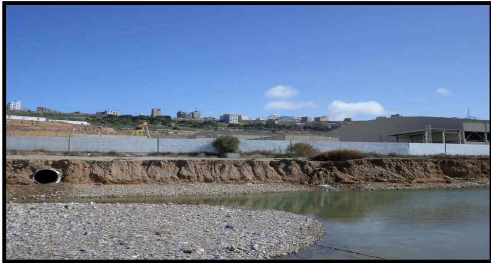
Figure 57 - Station de Pompage Souk Thlata
