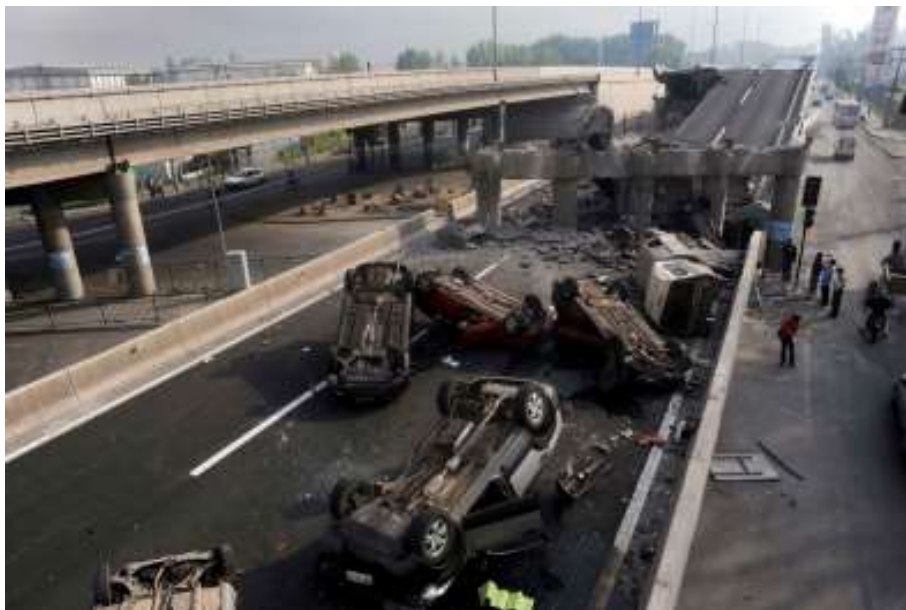
Figure I.4: Echappement d'appui au Chili 2010 (D. DAVI et al, 2013)
