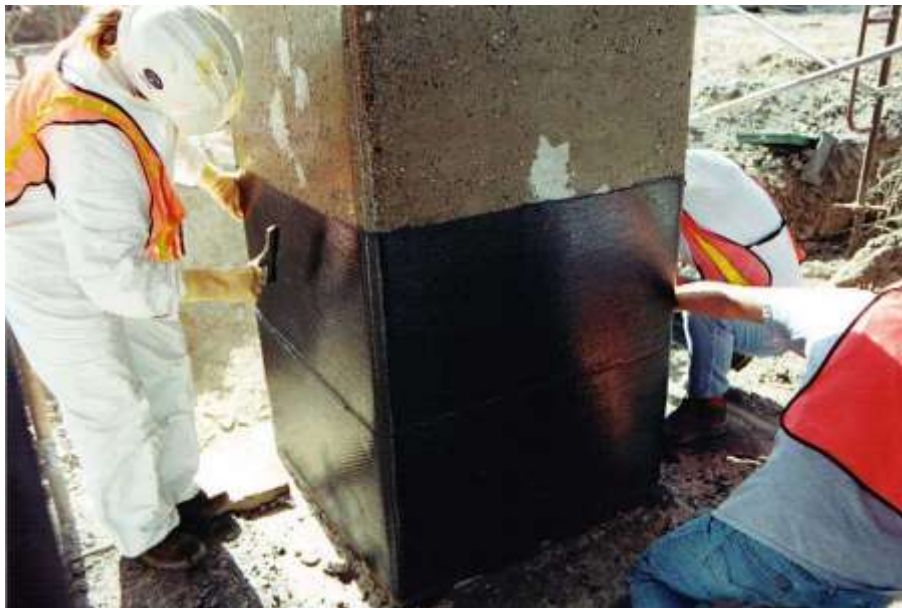
Figure II.14: Confinement de colonnes (Pantelides et al. 2002)
