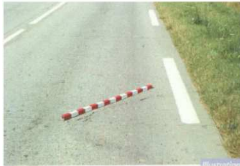
Figure 1.21 : Fissure oblique
