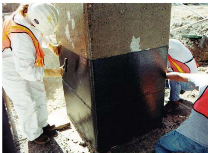
Figure IV.9: Confinement de colonnes [90]
